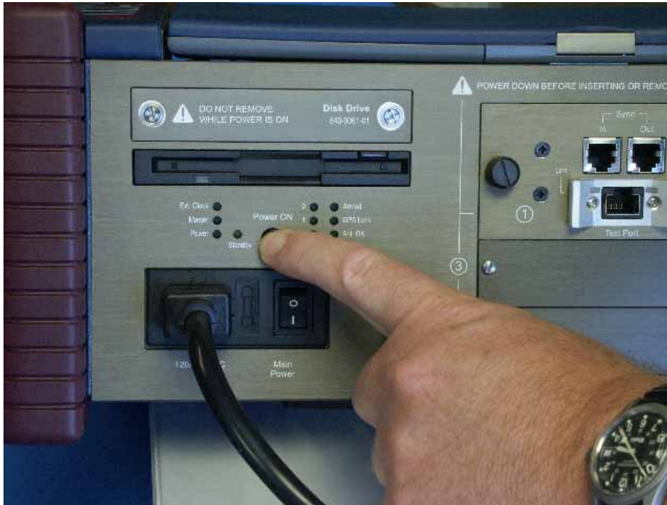
Figure 12-8. IXIA 250 Standby Switch
